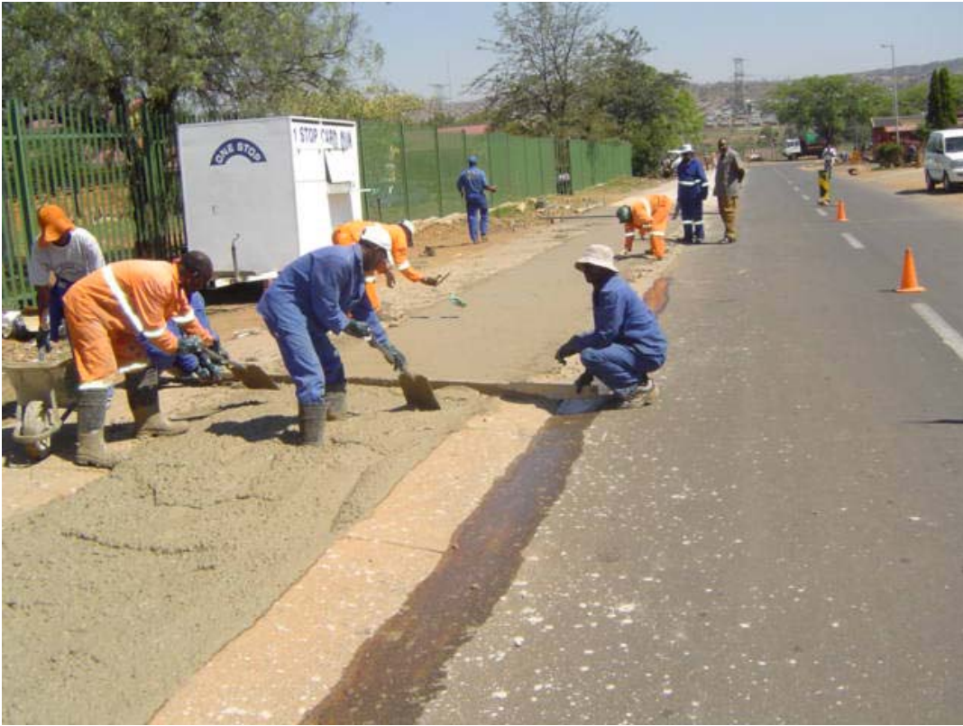
Figure 5: Labour-intensive construction of walkways
